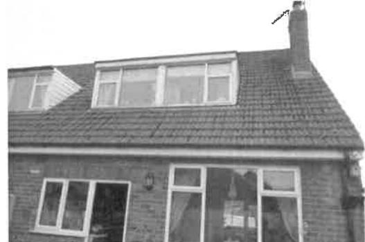
The roof consists of tiles with a bituminous roofing felt present. The loft space is well insulated and the loft space is illuminated and used for storage.
