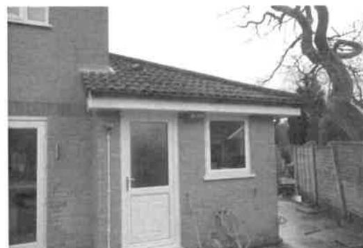
The roof consists of tiles with a bituminous roofing felt in good condition present. The loft space has some rock wool insulation.
