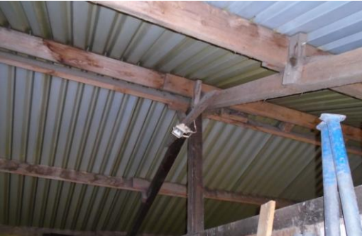
The roof structure is small section timber trusses and purlins they are relatively new timbers in good condition, which do not provide any potential bat habitat.
