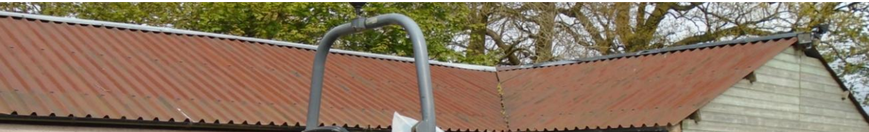
The roof is a simple L shaped pitch covered with profile steel sheet.
