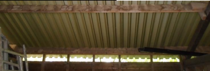
The steel sheets are in reasonable condition with most laps tight fitting. The only access points being at the eaves and gable abutments with the wall.
