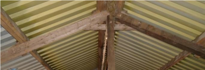
The roof structure is small section timber trusses and purlins they are relatively new timbers in good condition, which do not provide any potential bat habitat.
