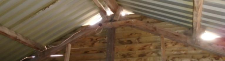
The steel sheets are in reasonable condition with most laps tight fitting. The only access points being at the eaves and gable abutments with the wall.
