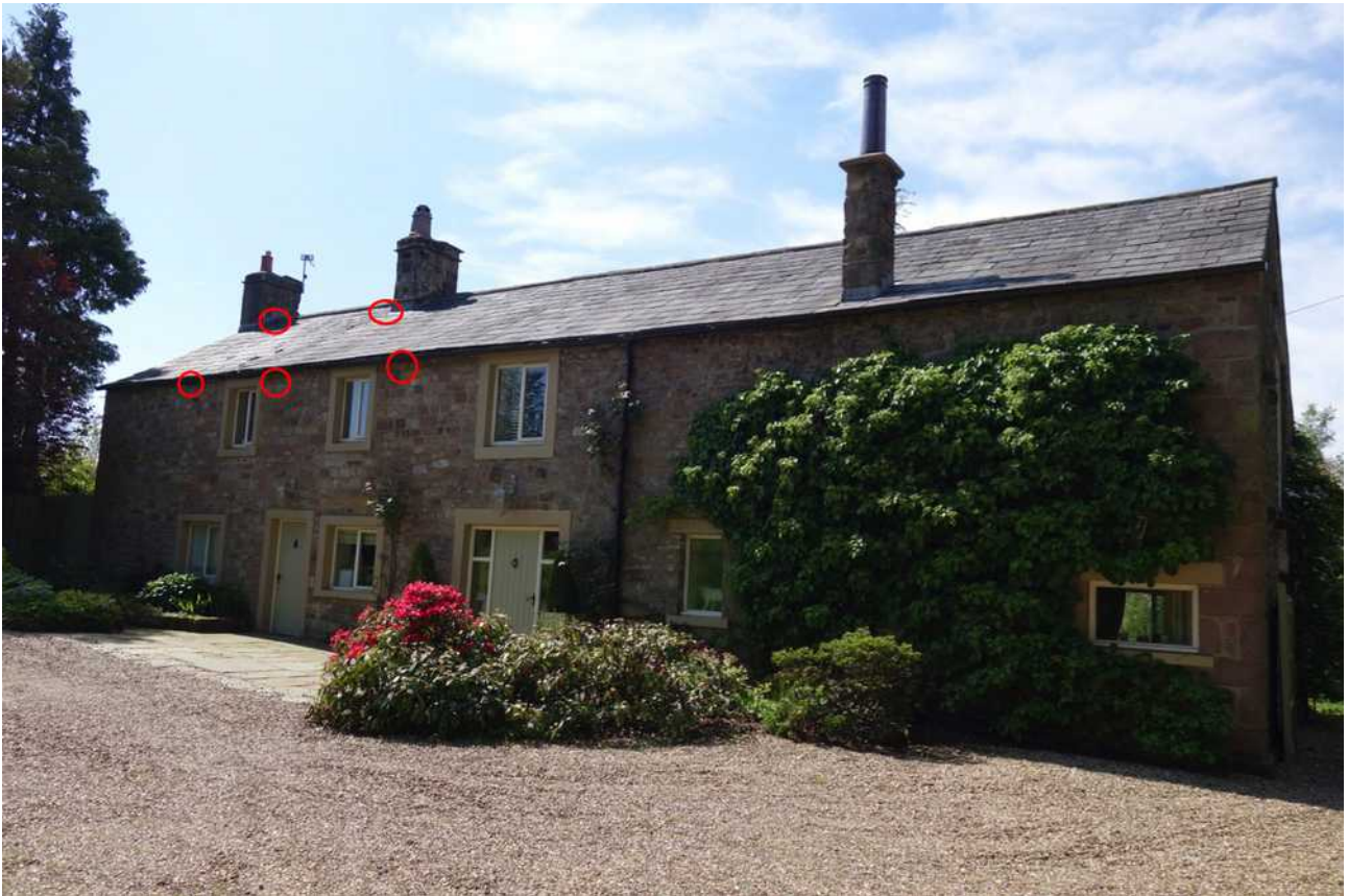
Brandt's bat roost entrances on north eastern aspect of roof.
