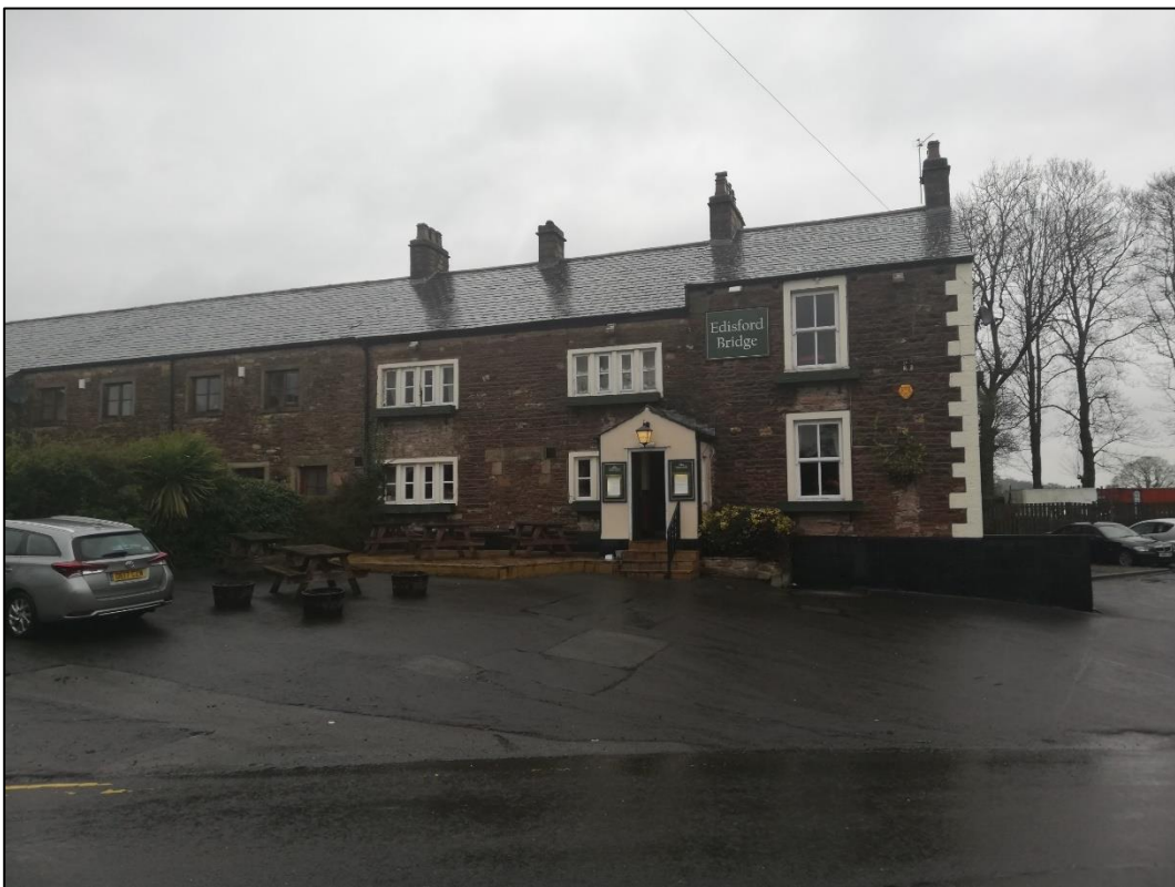
PL02: View north towards the Edisford Bridge Inn.
