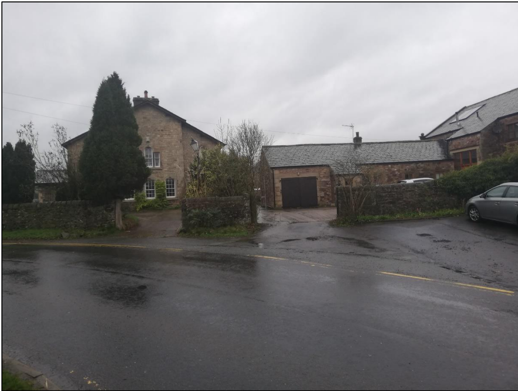
PL03: View west towards Edisford Bridge Cottage (left) and stable cottages (right).
