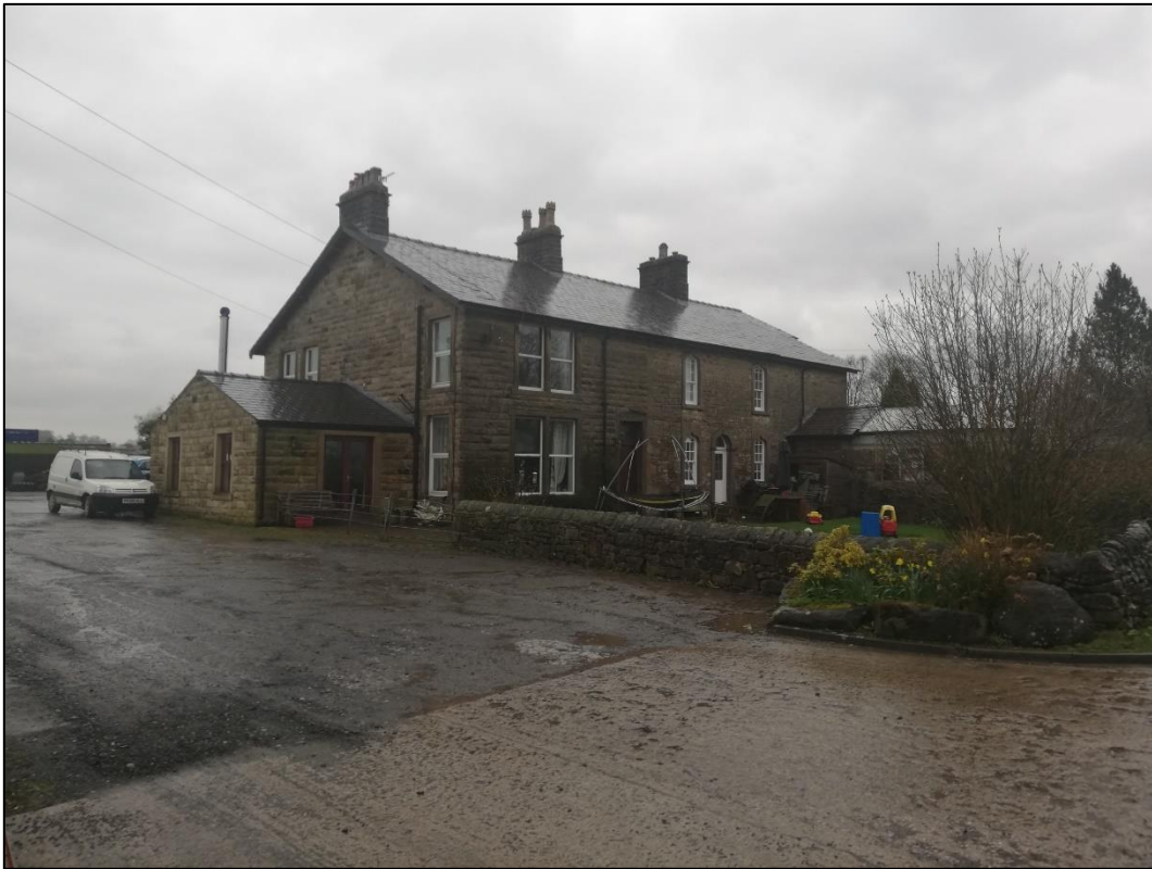
PL05: View north west towards Edisford Bridge Farmhouse and Cottage.
