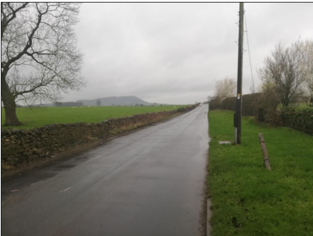
PL06: View west along Edisford Road.
