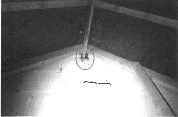
Roost entrance with droppings below.
