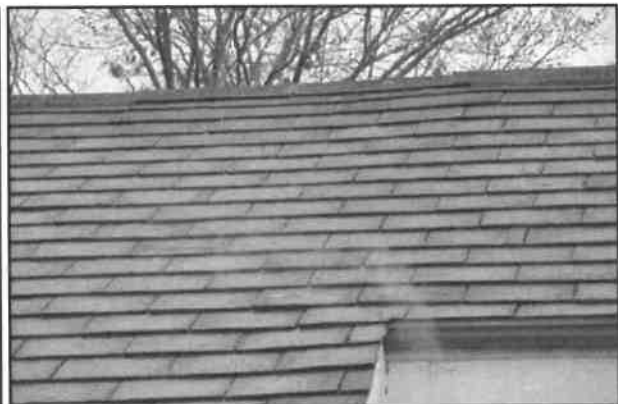
View of south gable, gaps are present along the roof edges (lhs) and view of main roof. There are gaps present along the ridge and between occasional lifted tiles (rhs).
