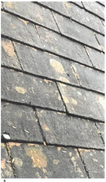
Image above shows cracked tiles and more patchy corroded tiles.
