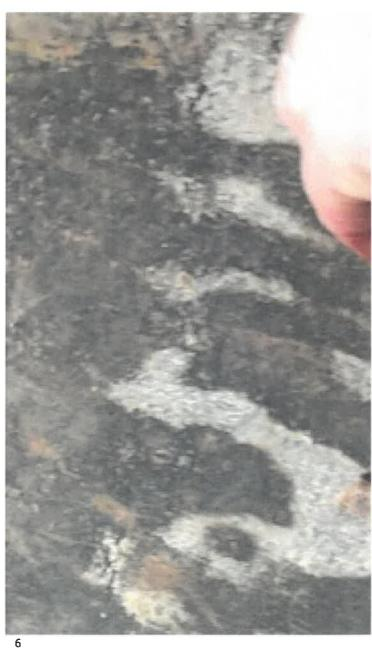
Image above shows how thin the roof tiles have become over time-the tile near my hand is the part that has been shielded from weather-the opposite end which is exposed is less than half the thickness so providing hardly any protection from the rain.
