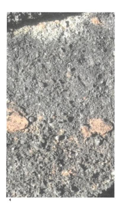
Image above shows corroded tiles which moss has damaged over time(the lighter colour shows the corrosion)
