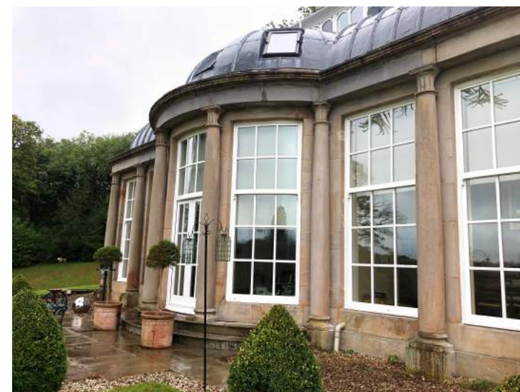
The front elevation of The Orangery
