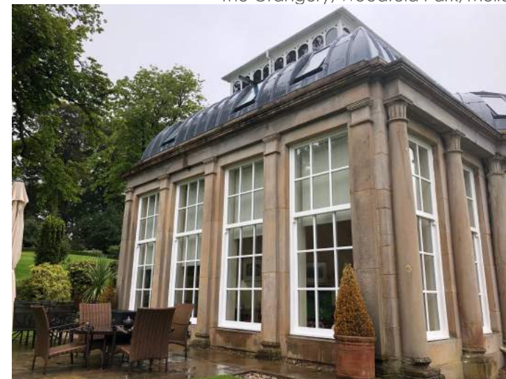
The West elevation of The Orangery
