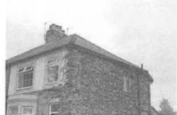
The property consists of a brick built semi detached two storey house with multi pitch slate roof. The first floor front wall and rear ground floor is rendered. A single storey single pitch roofed extension is present to the rear. Roofs feature well sealed ridge tiles and close fitting slates. Lead flashing is in good condition and close fitting.
