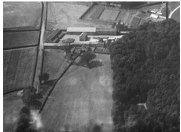
Plate 13 Aerial view of the farm, looking northwest, 1925 © Britain from Above, EPW013897
