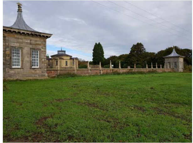
Plate 5 Garden wall and pavilions, looking north
