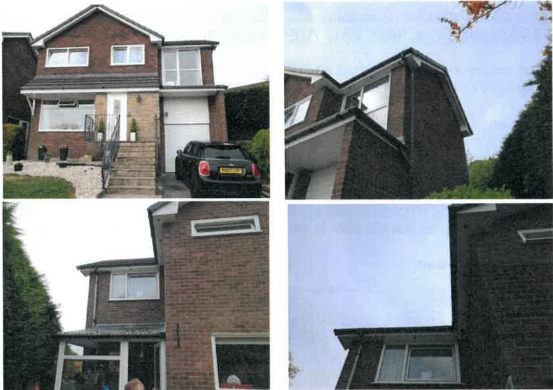
The property consists of a modern brick built detached house with multi pitched tiled roof. External walls are in good condition and well pointed with well sealed gables. Roof slates are close fitting with no lifted or missing slates, the ridge is well sealed and flashing where present is close fitting. Upvc soffits and fascia boards are close fitting with no gaps or crevices present.
