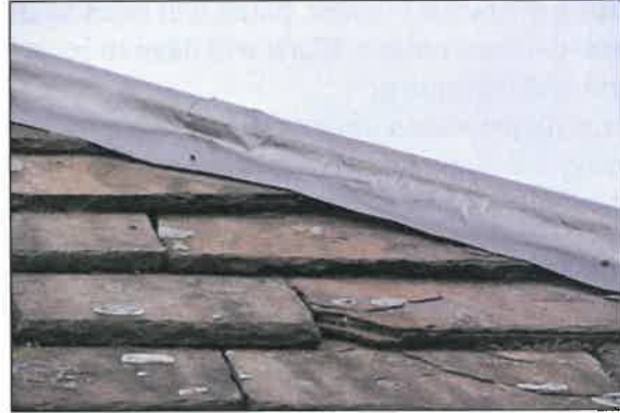
Image showing gaps along wall tops below roof overhang (lhs) and between stone tiles (rhs)
