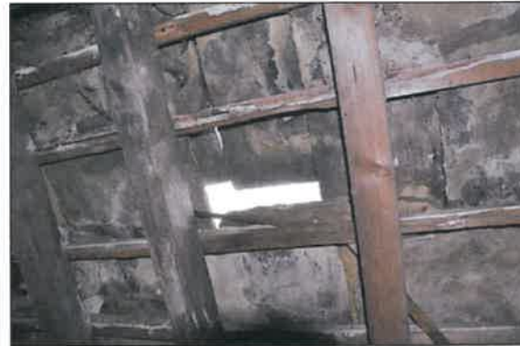
Image showing internal roof void with part intact torching (lhs) and gaps between the stone tiles (rhs)
