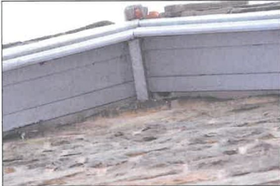
Image showing gaps along wall tops below roof overhang (lhs) and between stone tiles (rhs)
