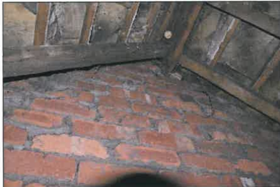
Image showing internal roof void with part intact torching (lhs) and gaps between the stone tiles (rhs)
