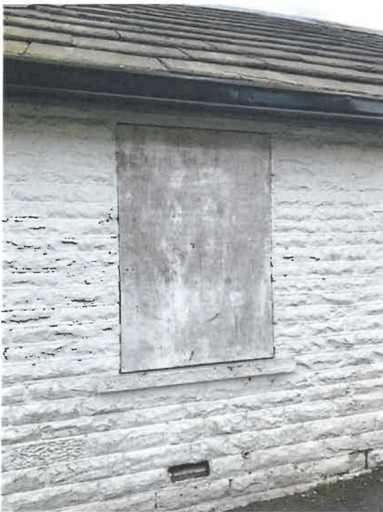
Image 2 shows the windows that are currently boarded up, it is proposed to protect the windows with roller shutters
