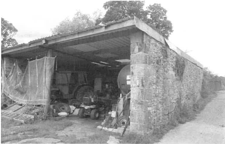
4 and 5 – An agricultural stone built lean to with single pitch corrugated roof used for storage and a modern single skin tractor store. The buildings offer low potential for roosting bats.
