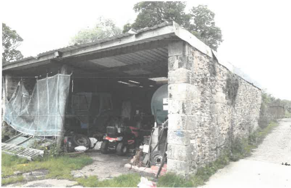
4 and 5 – An agricultural stone built lean to with single pitch corrugated roof used for storage and a modern single skin tractor store. The buildings offer low potential for roosting bats.
