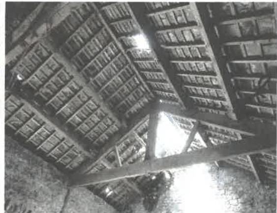
3 - A traditional stone built and slate roofed barn. Gaps and crevices are present in the external and internal walls. Roof slates are unlined and lifted tiles and missing tiles present. The building can be considered of high potential for roosting bats.
