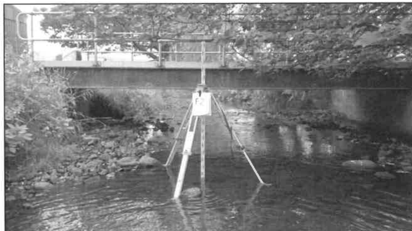
Figure 3-5: Bridge to Chipping WWTW
