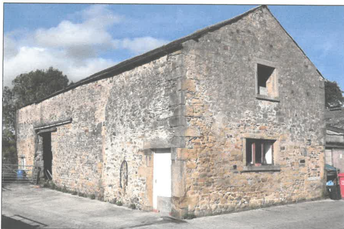
Photo 11 Barn: 19th century addition, east end
