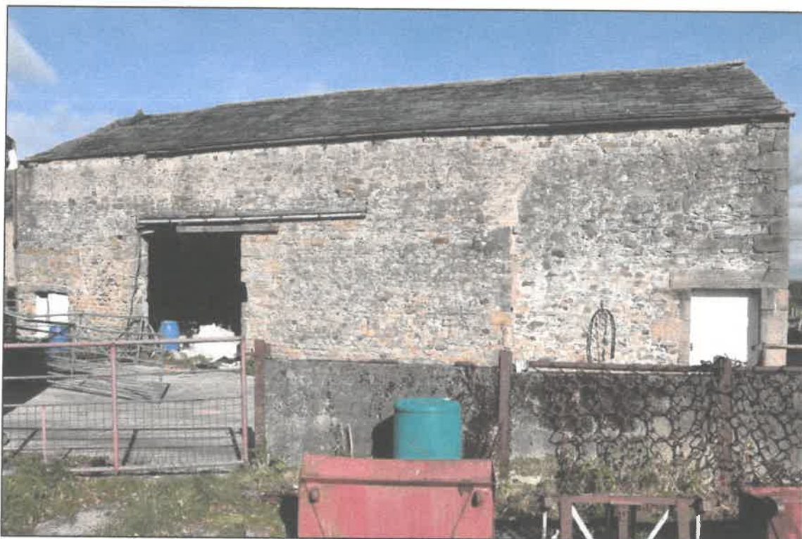
Photo 10 Barn: south front
