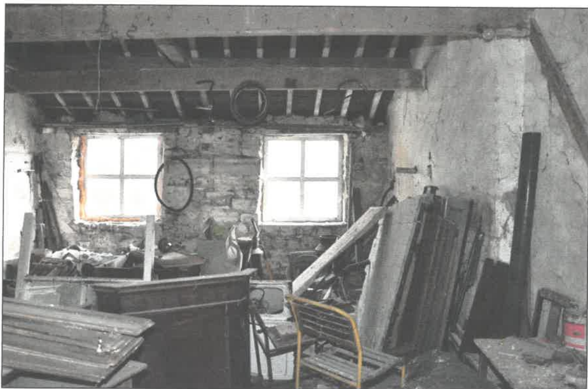
Photo 9 Garage/trap house: first floor, latterly joiner's workshop
