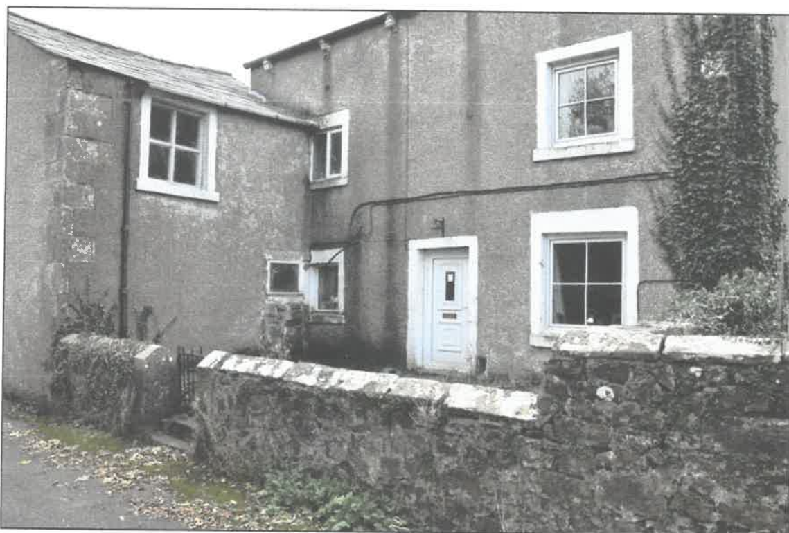
Photo 4: Farmhouse: rear elevation, with adjoining garage/trap house at left
