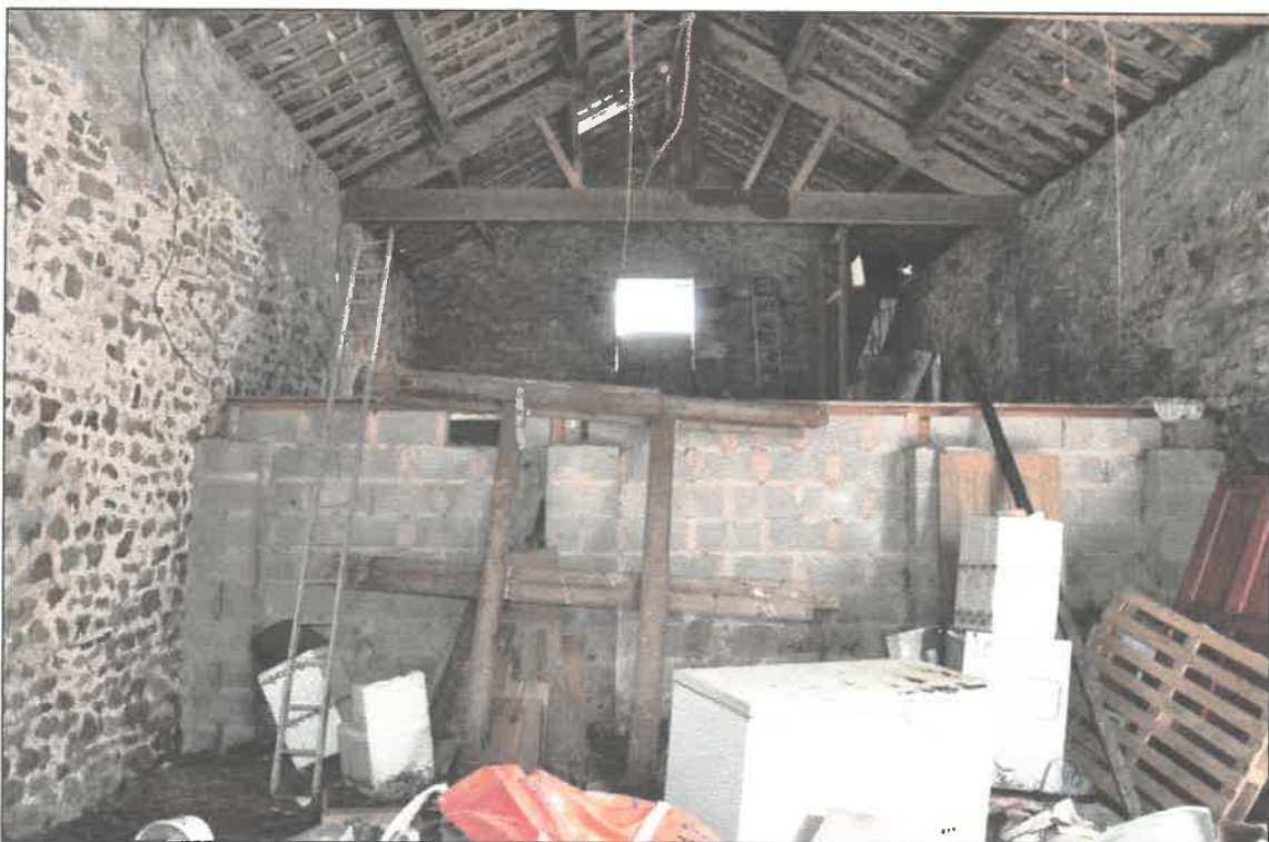
Photo 13 Barn: blockwork enclosing ice-creamery, east end
