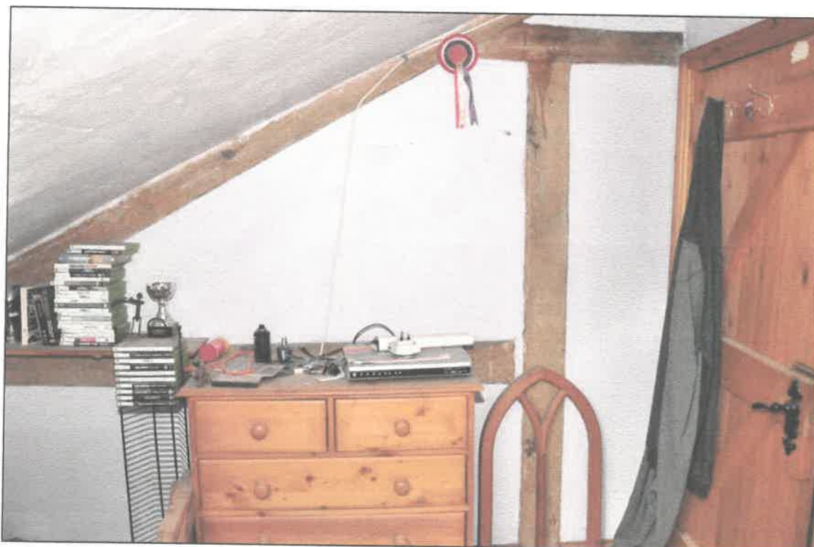
Photo 7: Farmhouse: roof truss forming partition on attic floor
