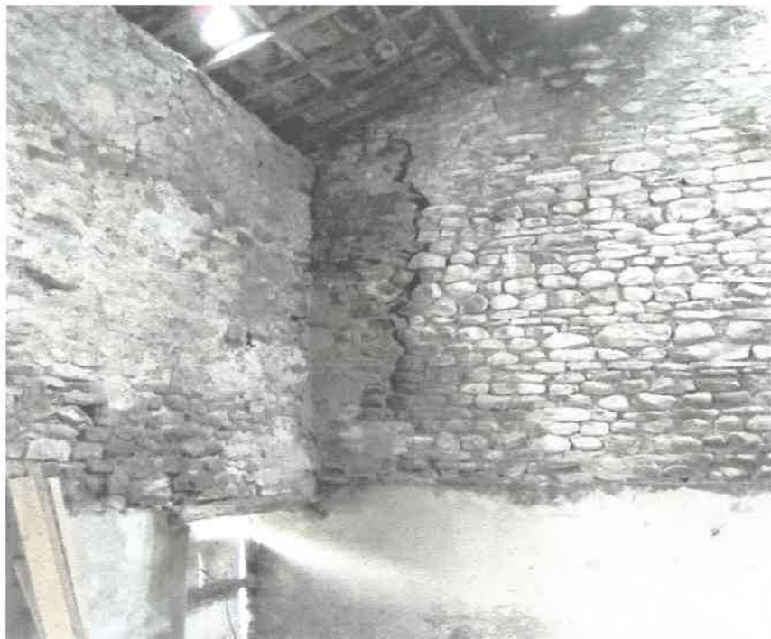
3b : Photo of West gable (Internally)
