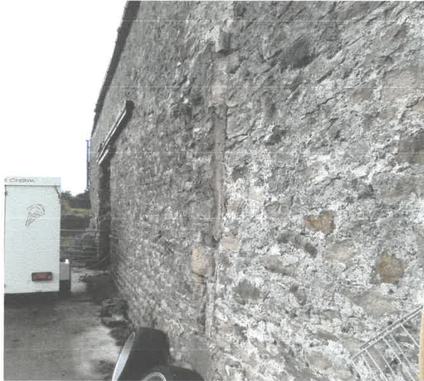
2a : Photo of Step in front elevation masonry
