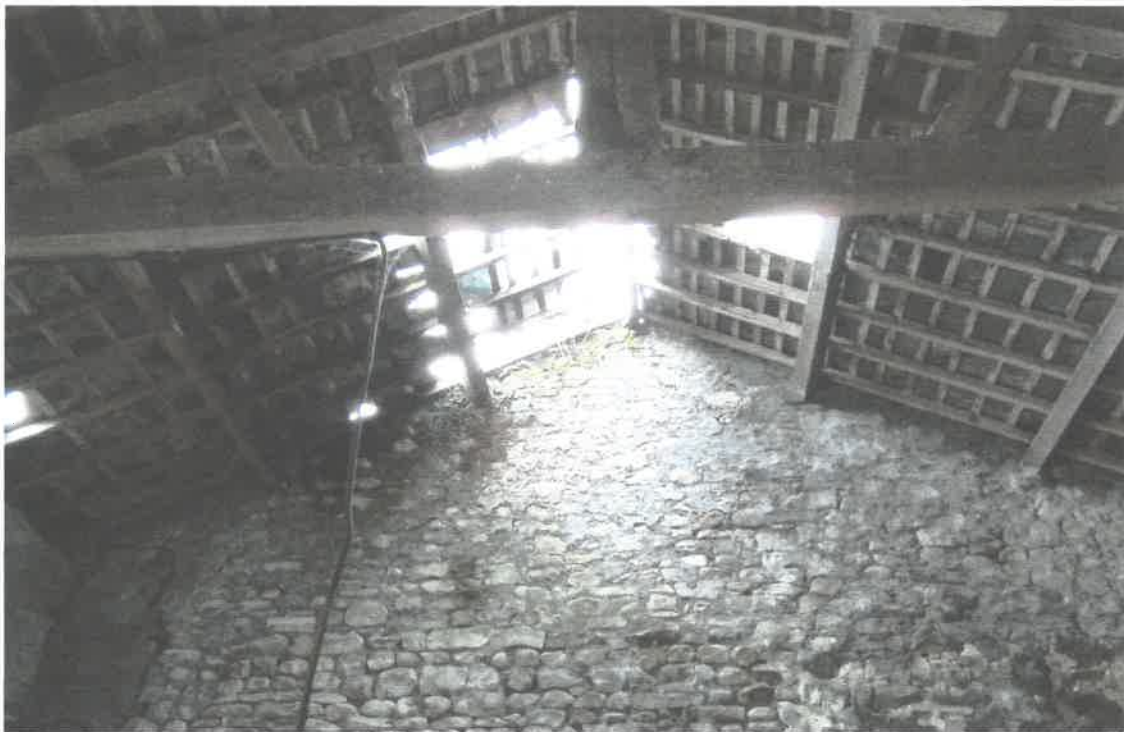
5a : Photo of internal roof structure -- East gable end
