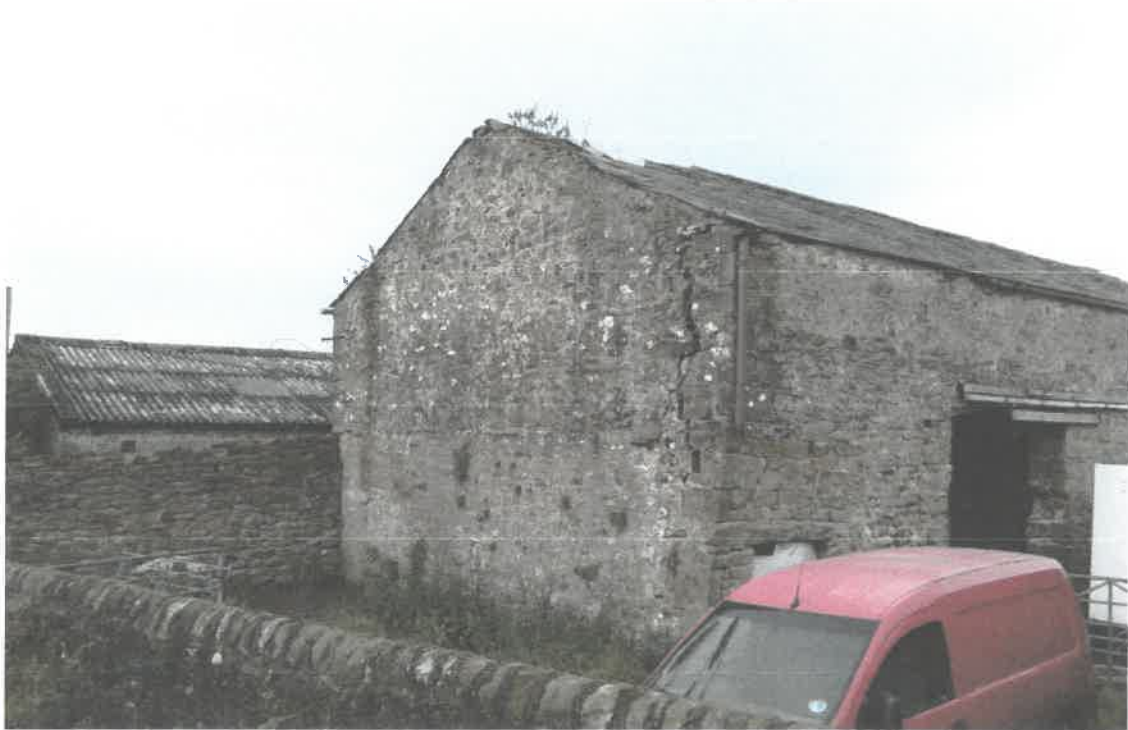
3a : Photo of West gable.
