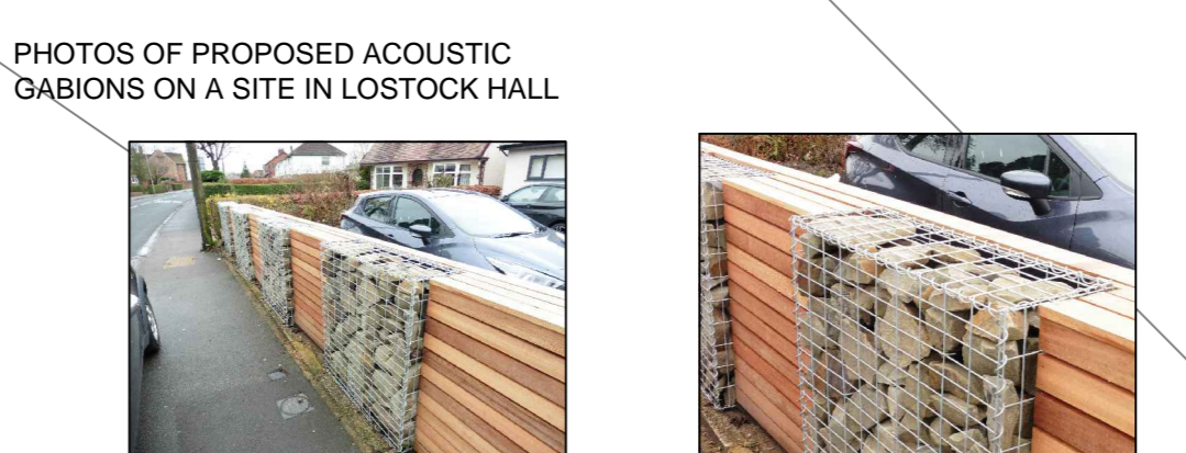
PHOTOS OF PROPOSED ACOUSTIC GABIONS ON A SITE IN LOSTOCK HALL
