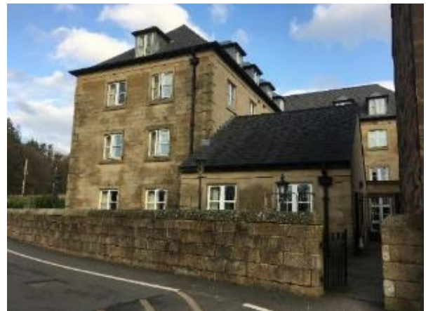
Figure 10: Site photo of Weld House
