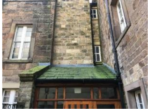
Figure 7: Site photo of lift tower
