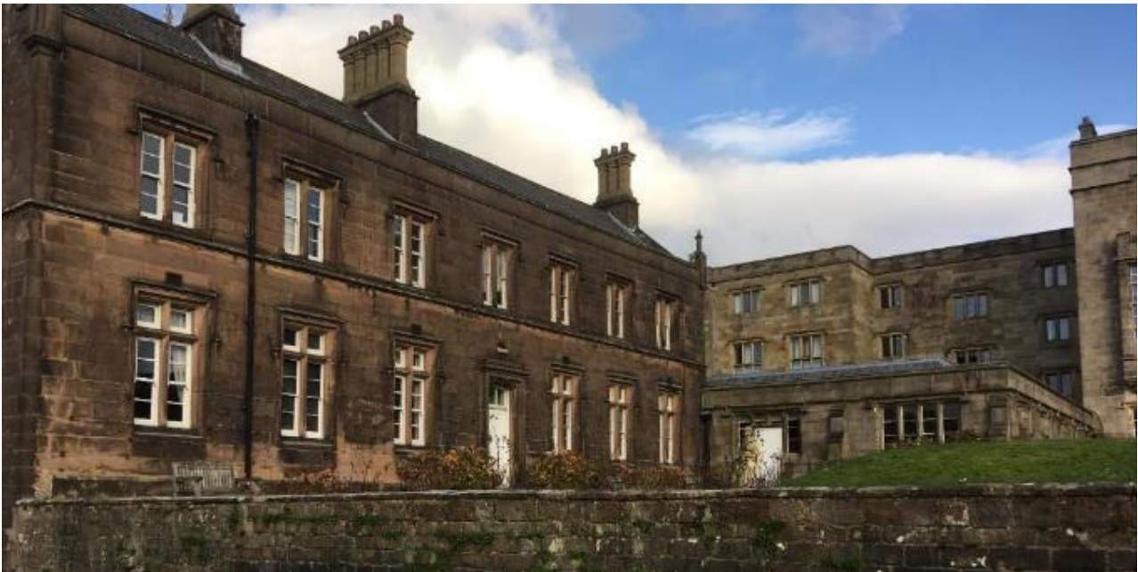
Figure 6: South elevation of Old Infirmary and link to main building
