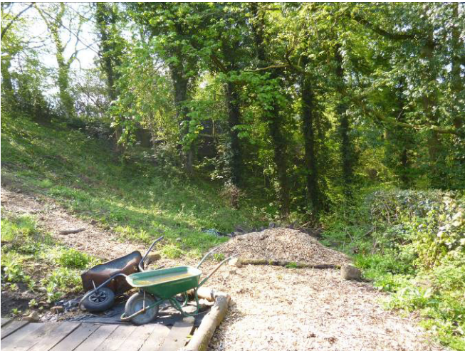
Looking into the SW corner of the site from the timber office.
