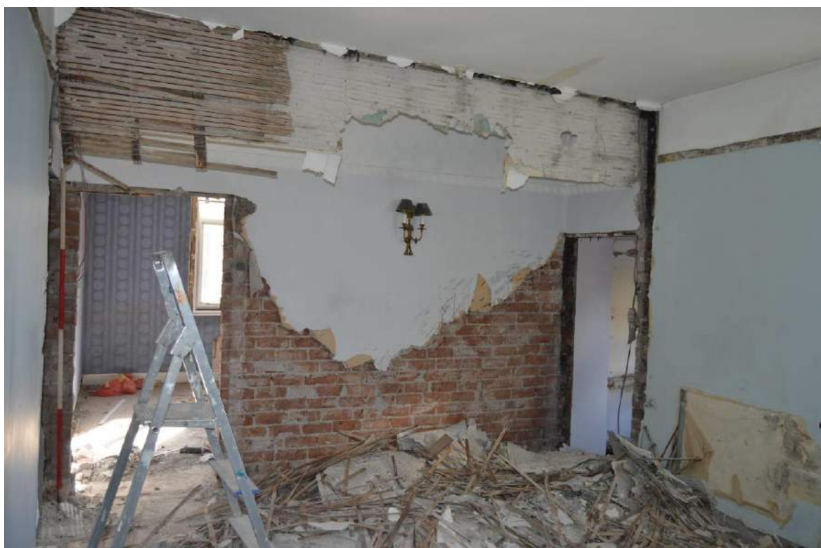
Plate 68: Interior of rear bedroom (F5). Note the lath and plaster dividing wall for the corridor (Scale: 1 x 2m).
