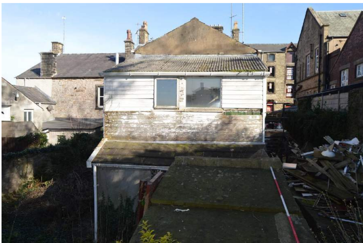
Plate 24: Rear gable wall of service range with timber frame projection (Scale: 1 x 2m).
