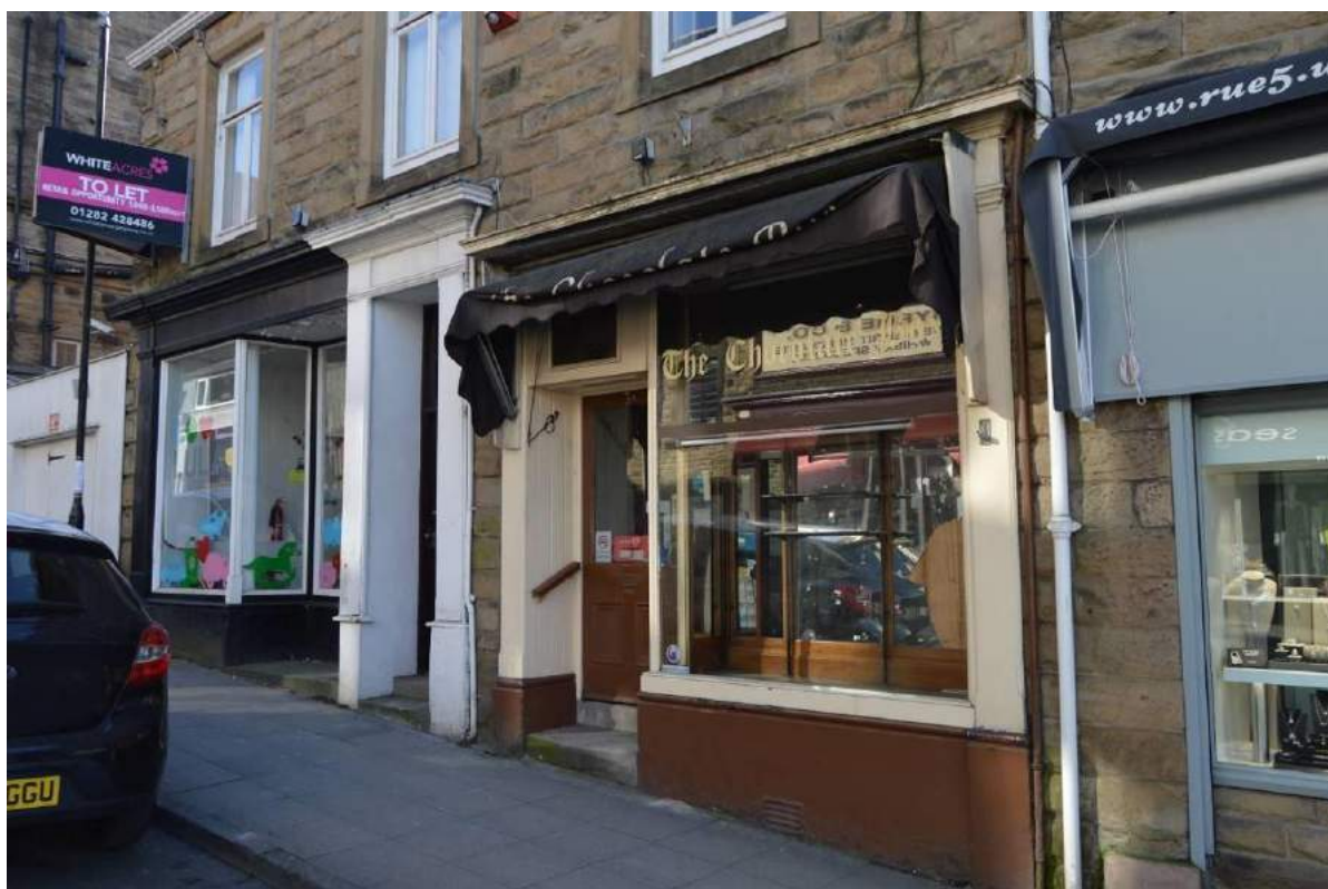
Plate 6: North shop front.
