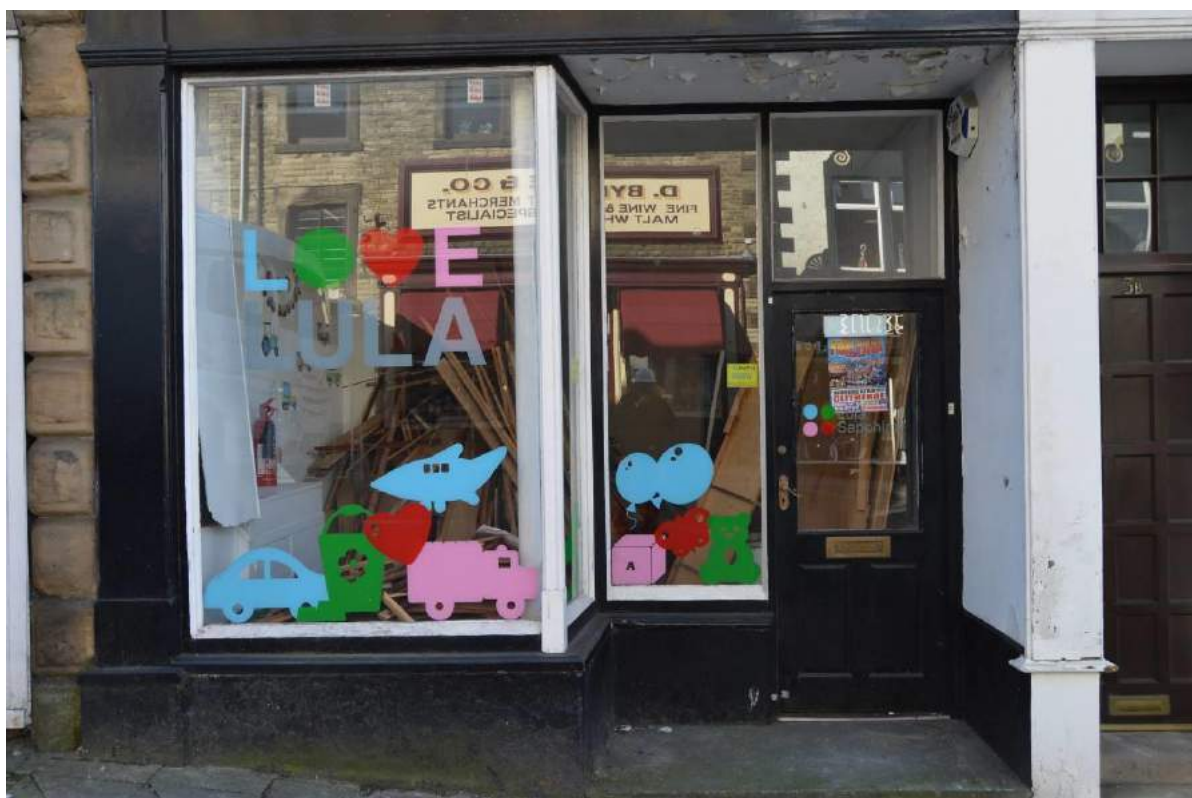
Plate 9: South shop front.
