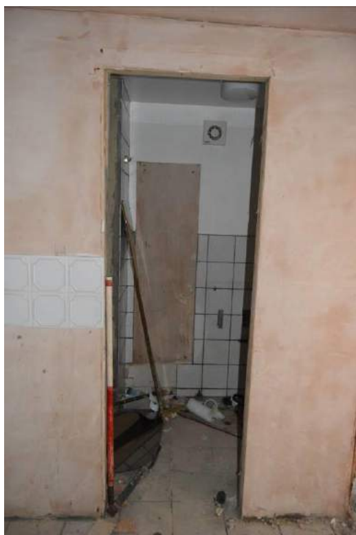
Plate 55: View inside pantry/bathroom (Scale: 1 x 2m).
