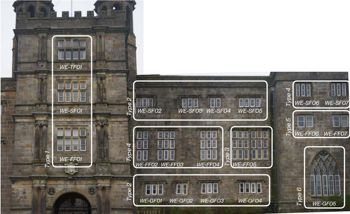
Photo of the West Elevation
