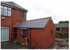
The roof consists of slates with plaster and lath present. A loft space is present in the main roof, it is insulated and partially boarded.
