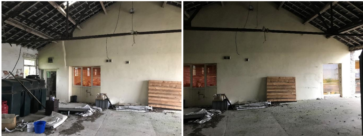
Rear view of Old Sawley Grange from within the rear shippin.
