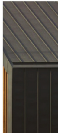
Aluminium grey metal cladding to roof and wall sections
