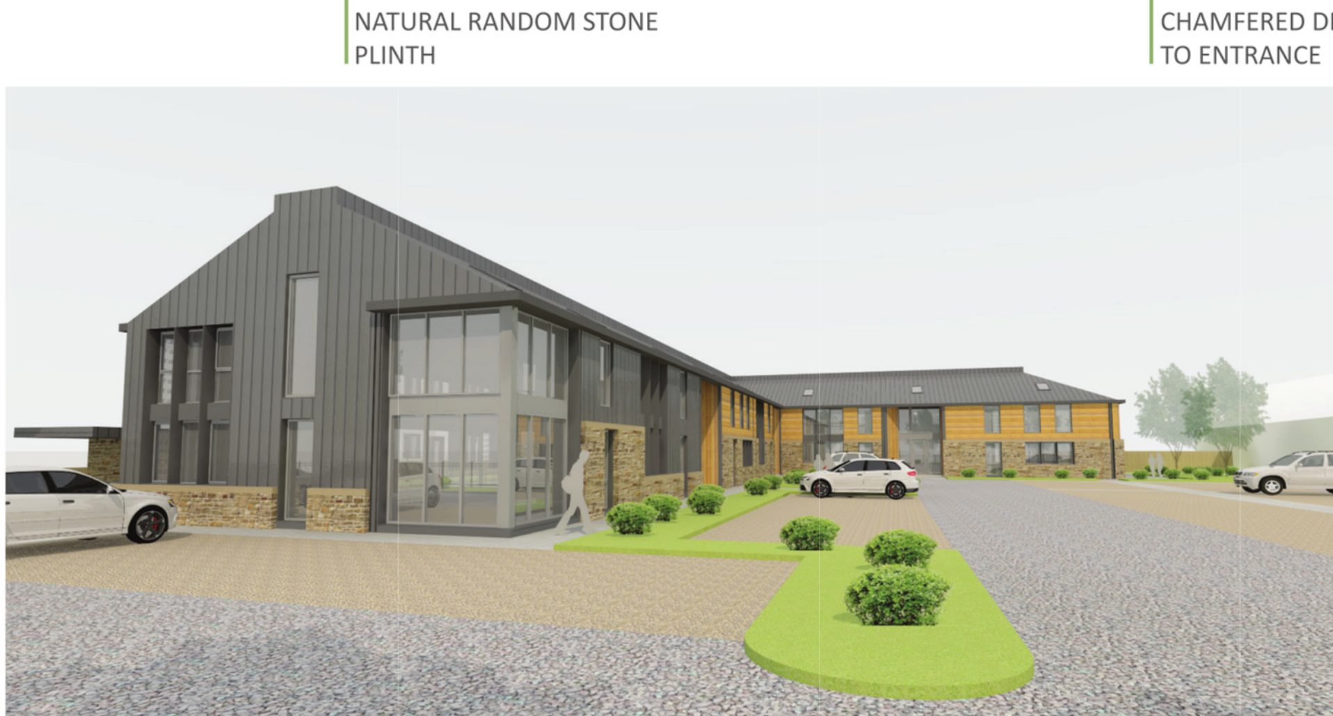
Aluminium grey metal cladding to roof and wall sections
