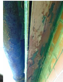
Eaves soffit to slated section
