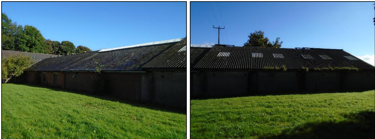
PL01: View of the outbuilding to be demolished (first phase to the left and second phase to the right).
