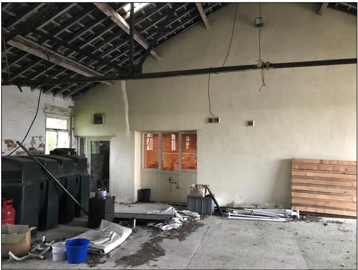
PL00: View north looking towards Sawley Old Grange from within the rear outbuilding showing the render wall finish.
