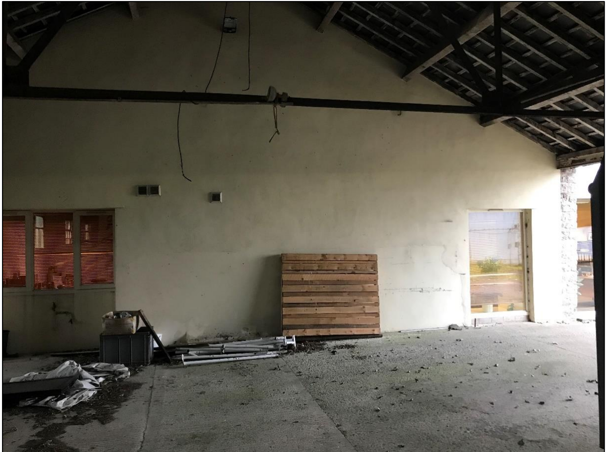
PL01: View north looking towards Sawley Old Grange from within the rear outbuilding showing the render wall finish.
