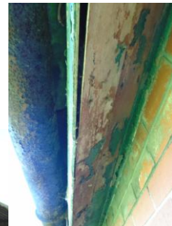
Eaves soffit to slated section
