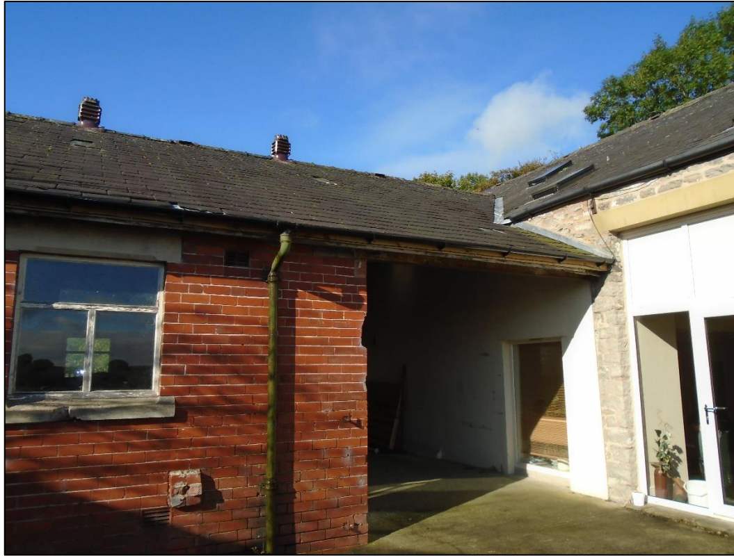
PL02: Junction between the rear south facing elevation of Sawley Old Grange and the adjoining outbuilding (to be demolished).
