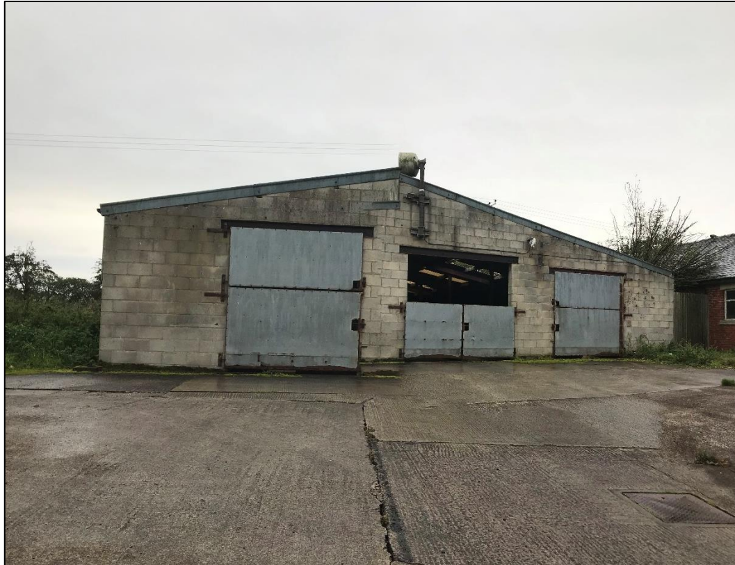
PL07: View of detached outbuilding to be demolished.
