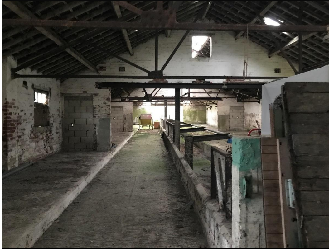
PL06: View south within the rear outbuilding.
