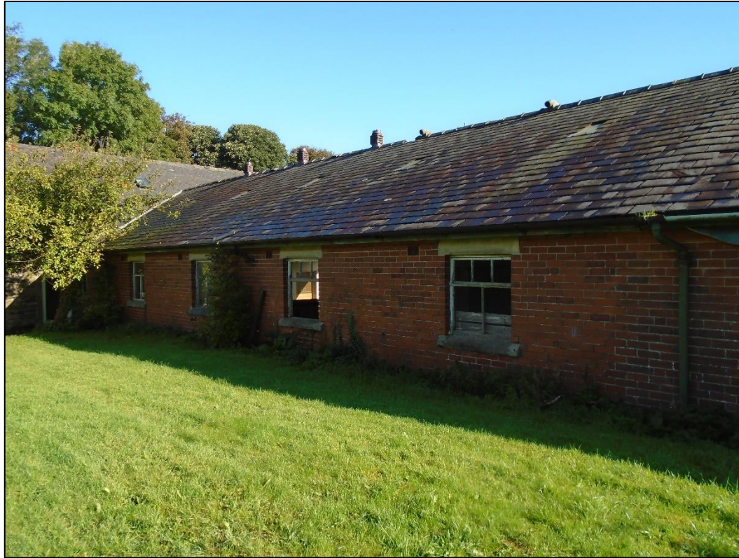
PL03: View of adjoining outbuilding (to be demolished) from the south west.
