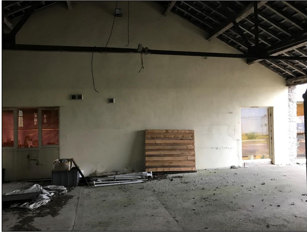
PL05: View north looking towards Sawley Old Grange from within the rear outbuilding.
