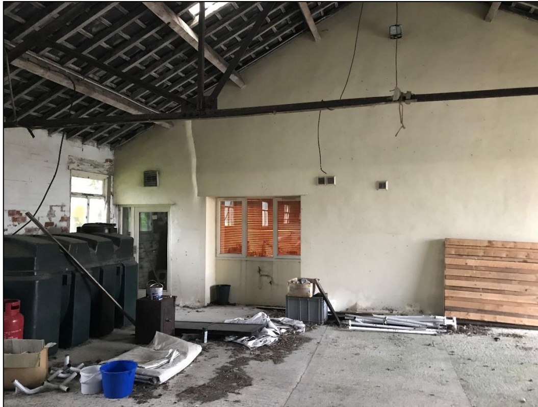
PL04: View north looking towards Sawley Old Grange from within the rear outbuilding.
