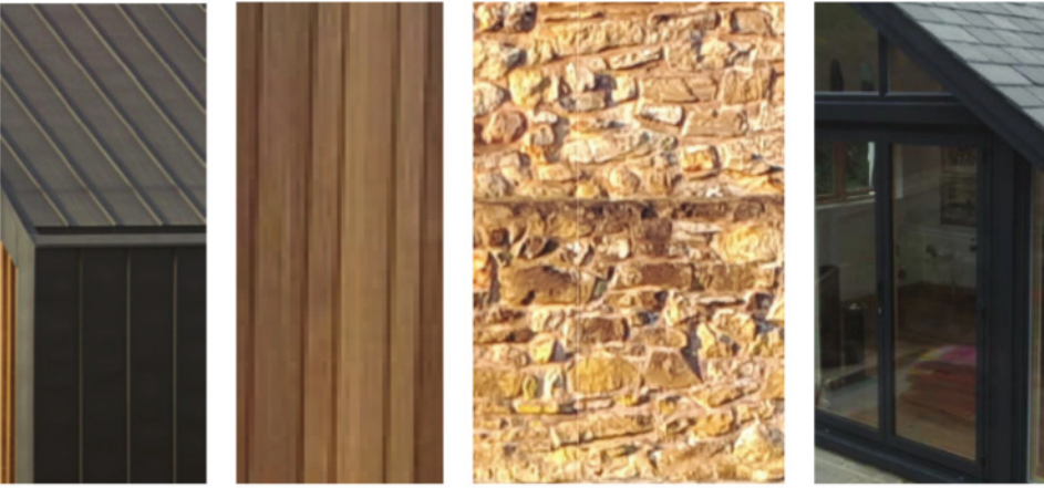
Aluminium grey metal cladding to roof and wall sections Timber cladding Random natural stone to match existing Grey Aluminium glazing
