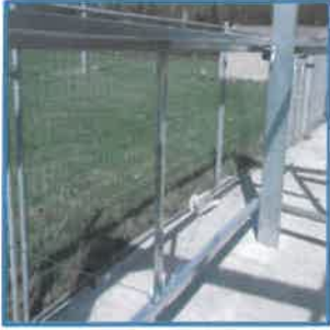
Anti-sag system as required by BS5950.
