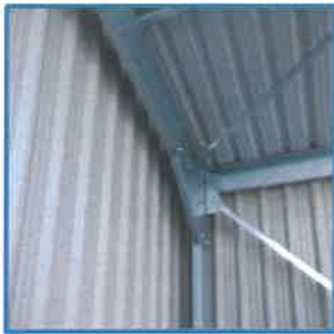
Anti-condensation lining on all single skin roof panels.
