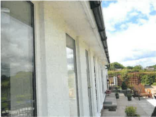
Rear northern elevation showing tight fitting fascias / soffits.
