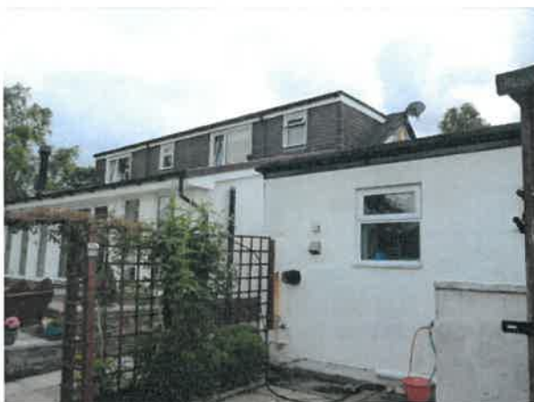
Rear northern elevation, general view. Showing existing flat roof garage with negligible bat roost potential.
