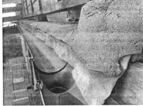
Photo 10: Layers of roofing materials, beam and gutter.
