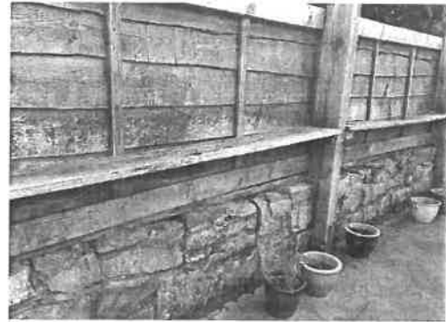
Photo 14: Timber fencing and stone wall boundary (height extended on the northern boundary)
