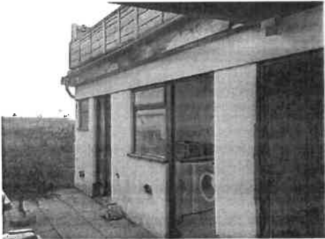
Photo 7: Ground level view of building exterior
