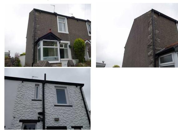
The property consists of a two storey end terraced house with double pitched slate roof, a porch is located on the eastern facade with a double pitched slte roof. External walls are rendered with no cracks or crevices present.
