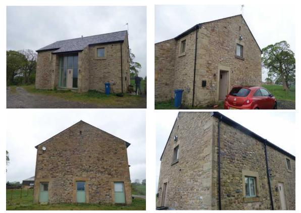
The property consists of a recently (2010) converted stone farmhouse with double pitched slate roof. External walls are in good condition and well pointed with well sealed gables. Roof slates are close fitting with no lifted or missing slates, the ridge is well sealed and flashing where present is close fitting. Fascia boards are close fitting with no gaps or crevices present.
