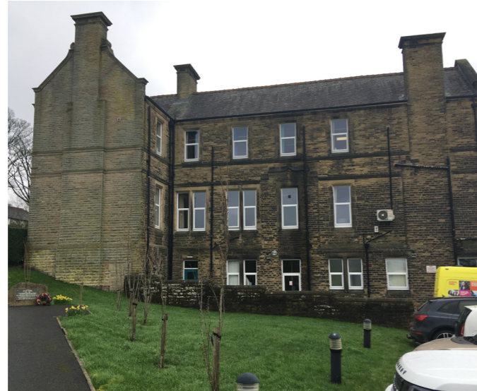
View from the car park of east elevation and memorial
