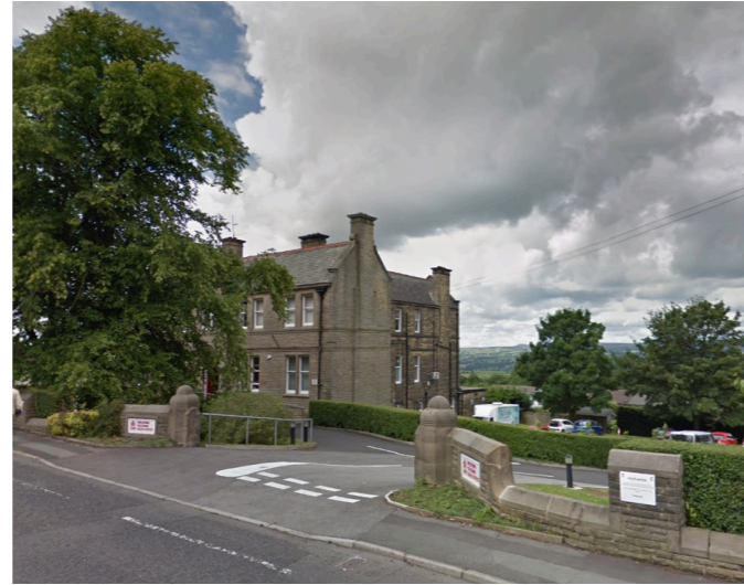
View from Whalley Road looking at East elevation.
