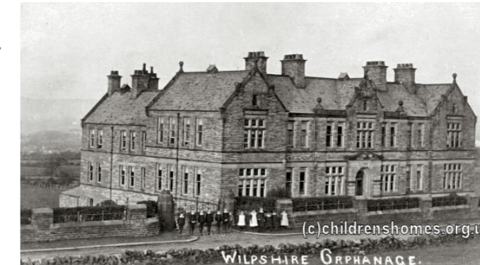
The original Orphanage building
