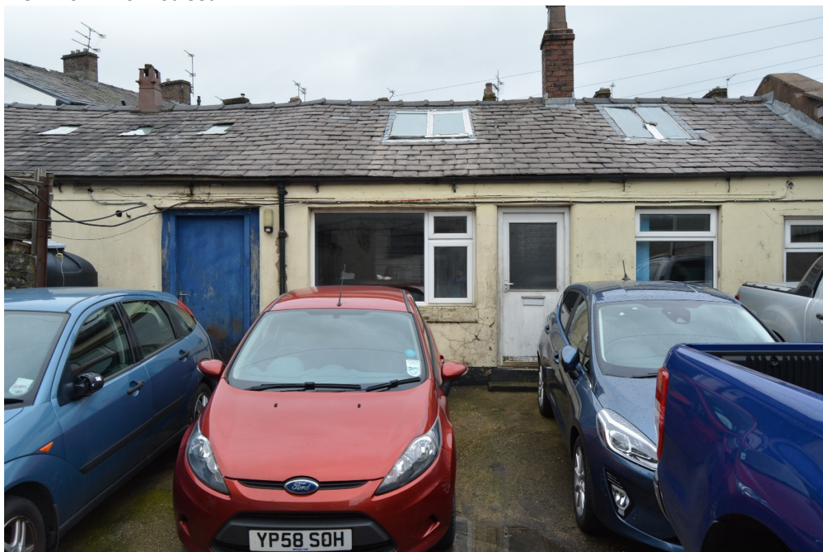
Existing Single Storey Building To Be Demolished
