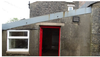
Figure 11: existing rear kitchen extension
