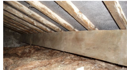
Figure 9: inside eaves void
