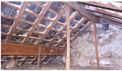
Figure 10: roof void, single story extension
