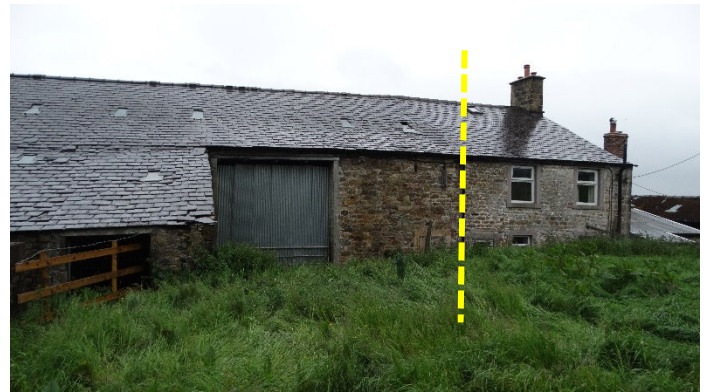
Figure 6: rear elevation barn (left) and farmhouse (right)
