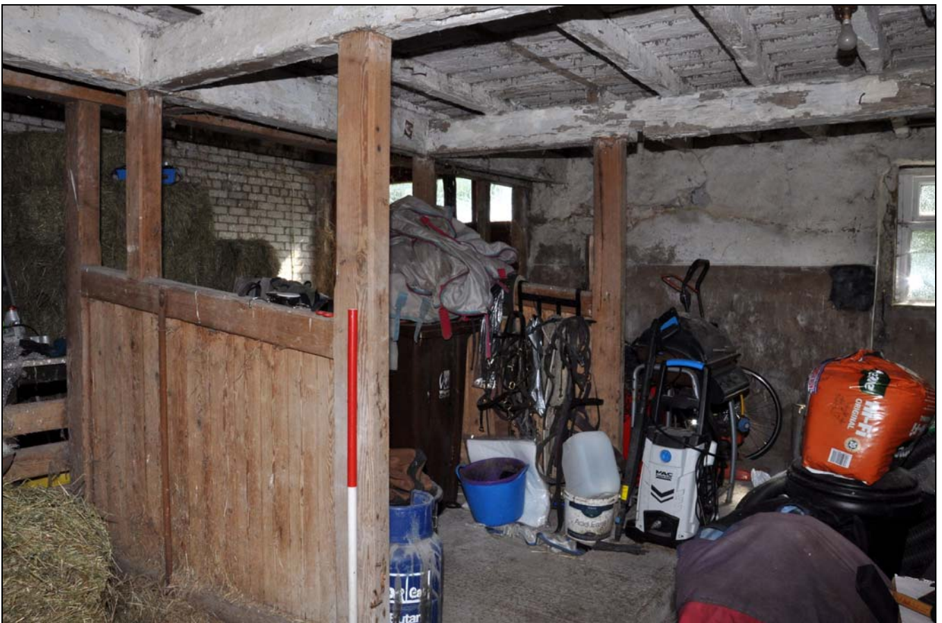
Photo 11: Stalls in shippon, looking east, showing later boskins and front beam to loft
