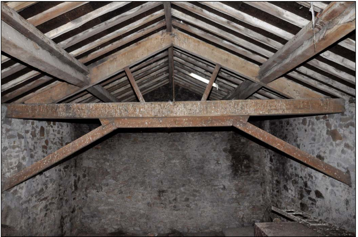
Photo 18: South-west truss, looking south-west
