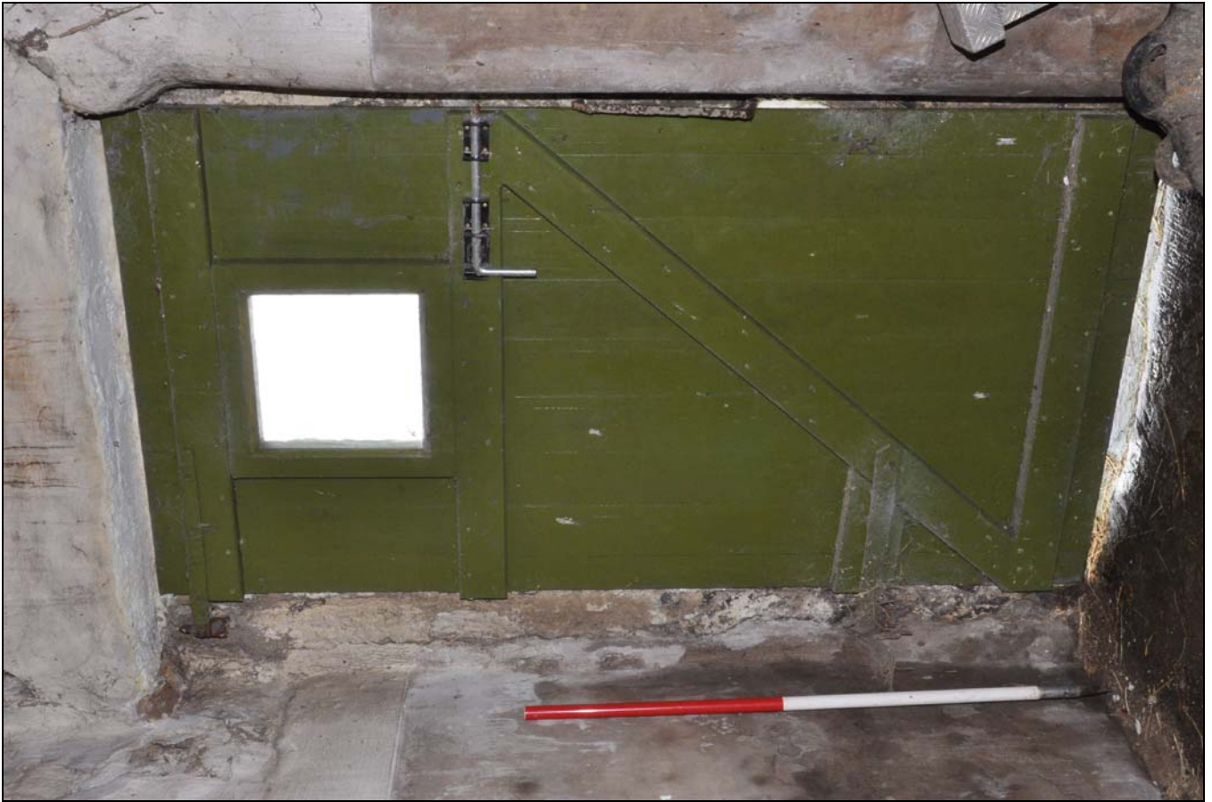
Photo 14: Detail of doorway in north-west side of shippon
