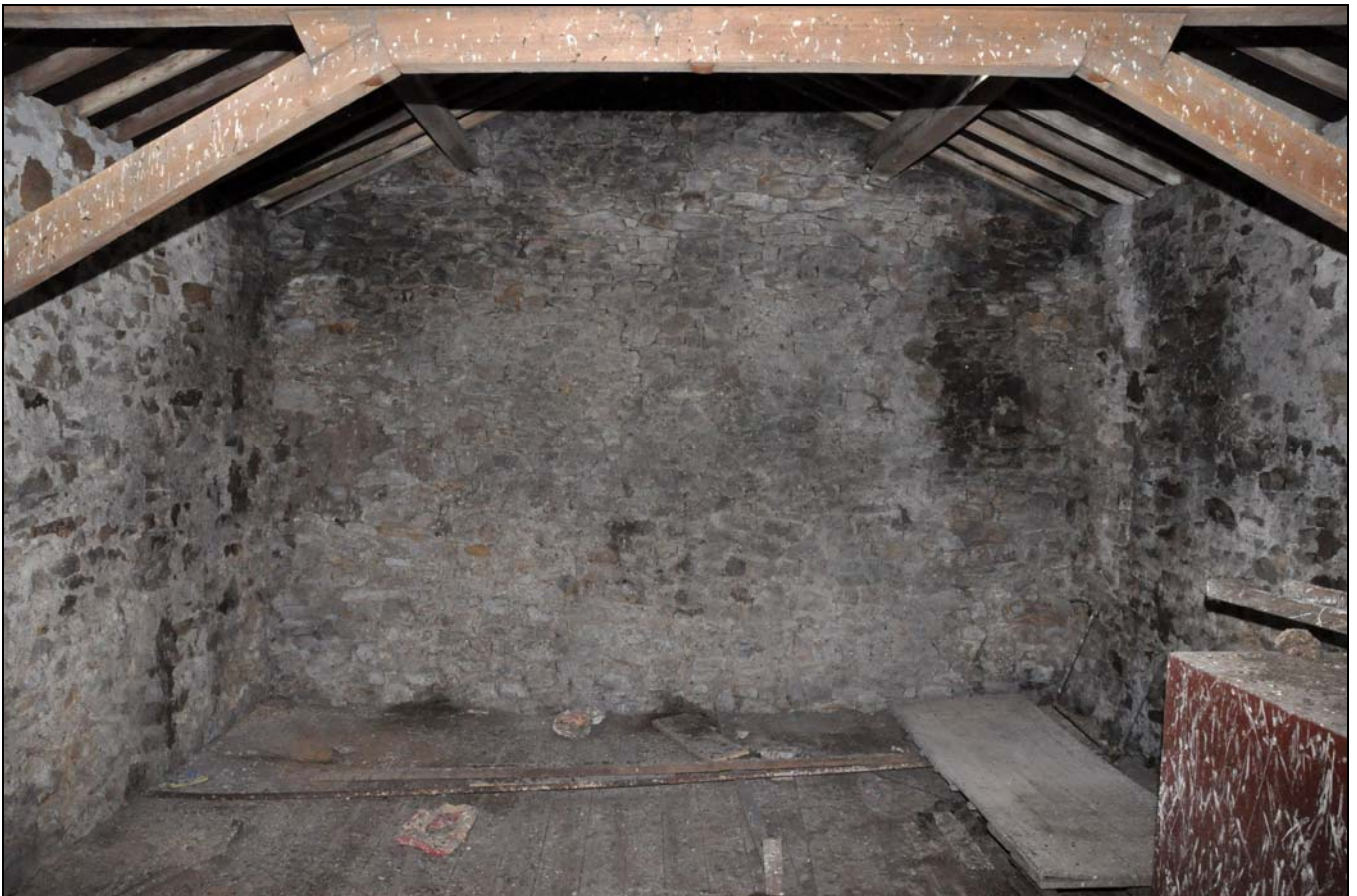
Photo 15: Hay loft over shippon, looking south-west
