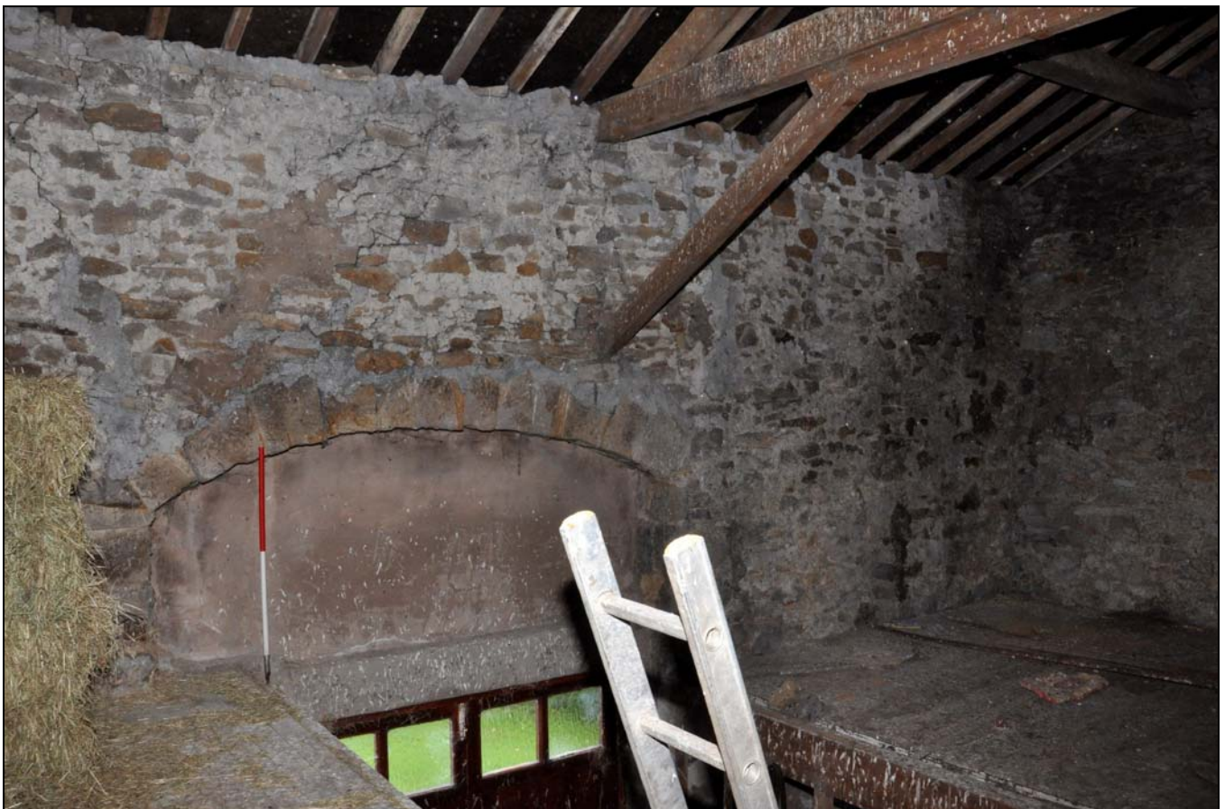
Photo 8: Interior view of front cart entrance, from the north
