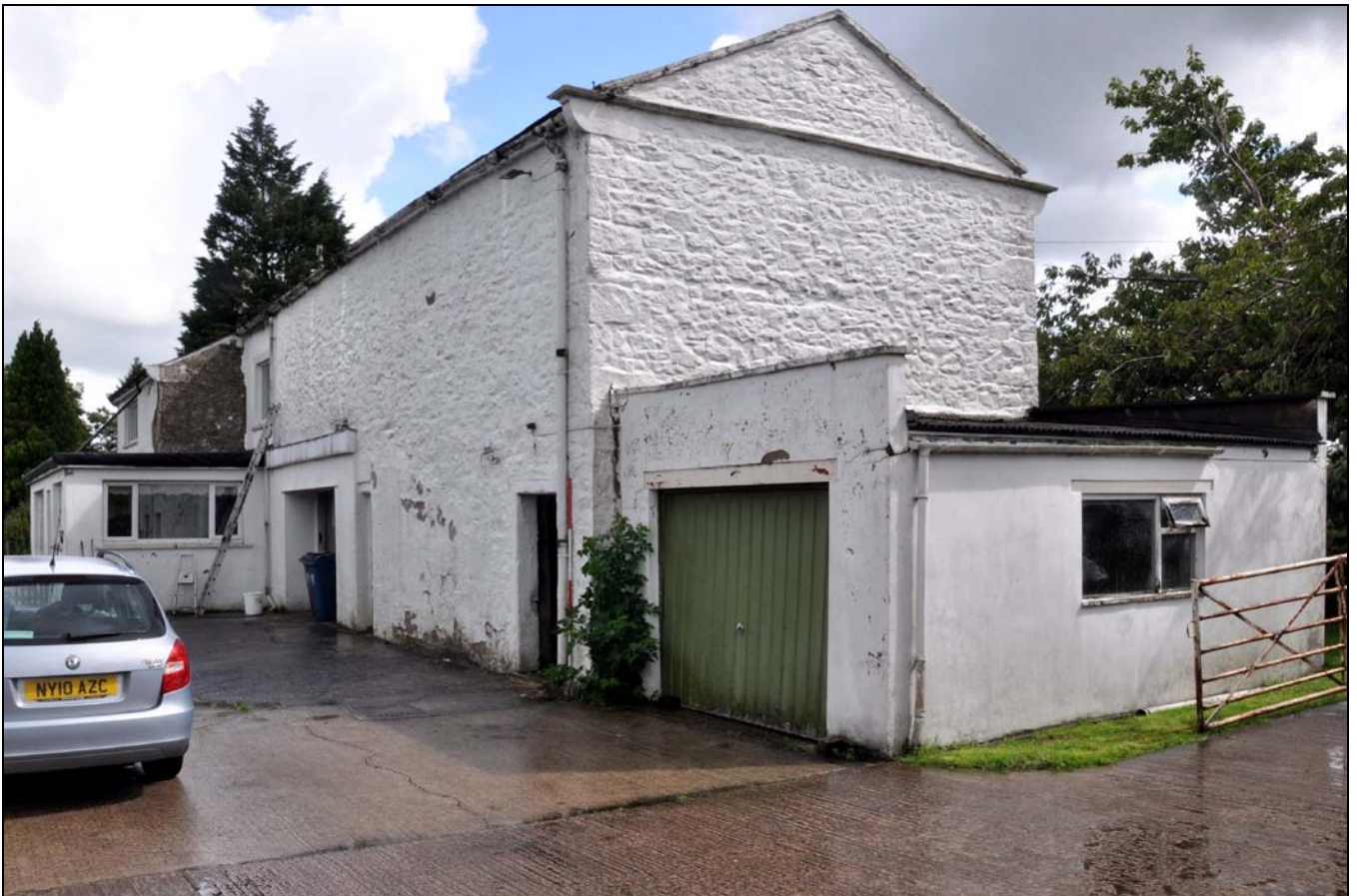
Photo 5: General view of the barn and house from the west
