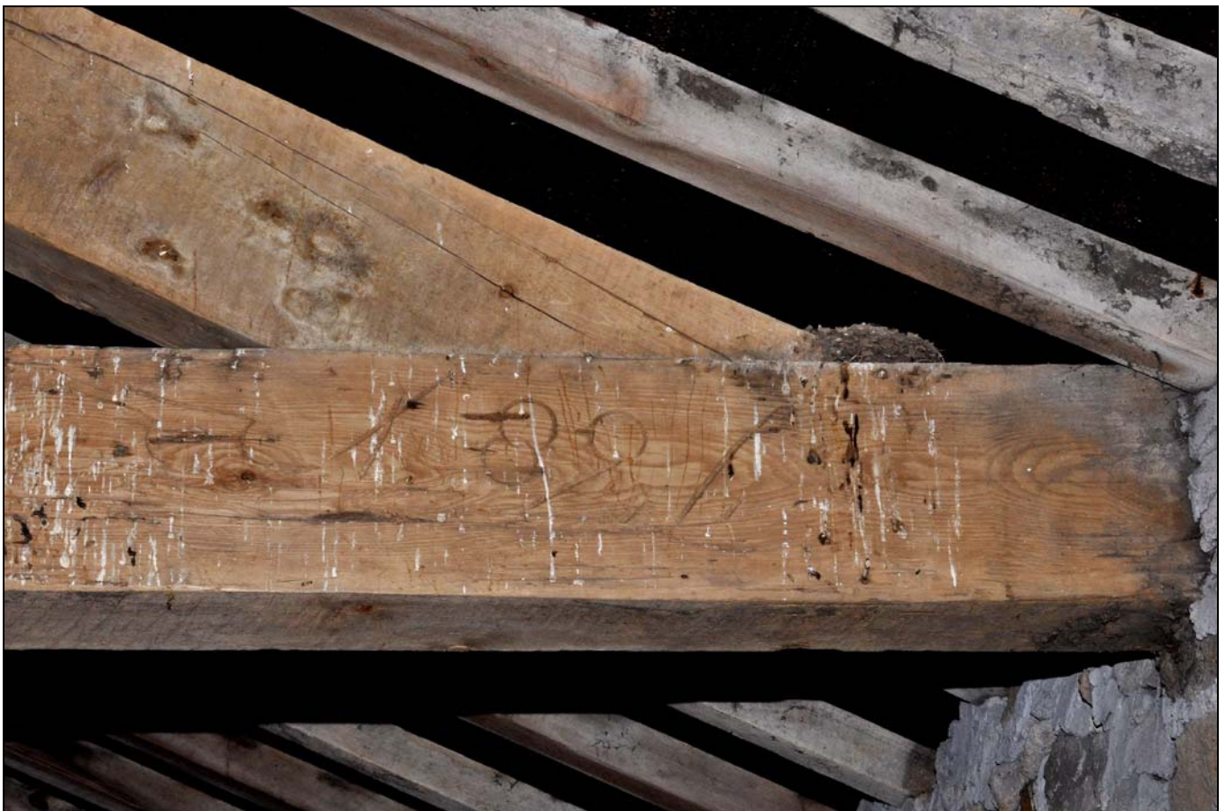
Photo 19: "Baltic" mark on north-east side of south-west tie beam
