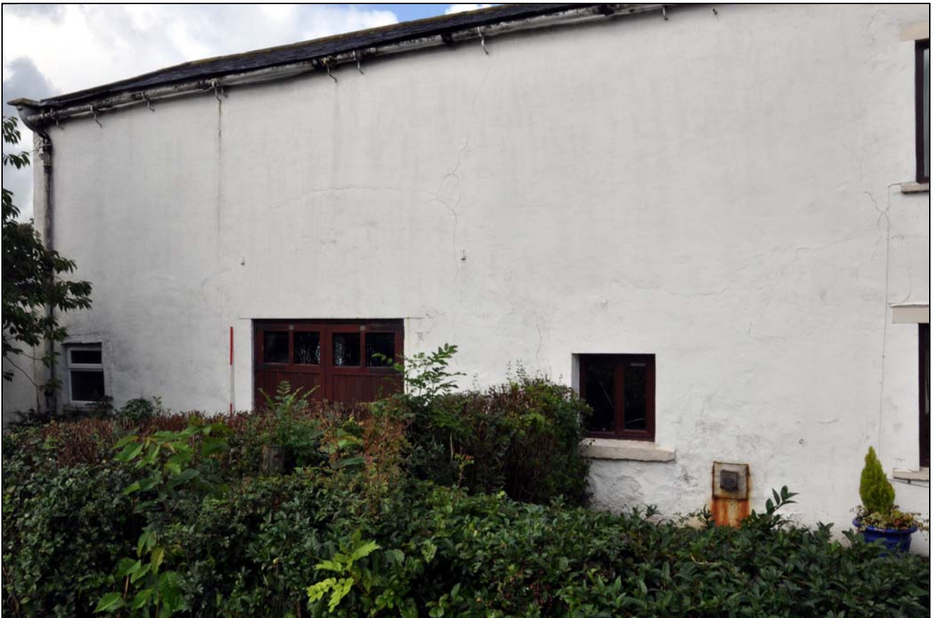
Photo 2: Front elevation of the barn, with traces of arched cart entry visible above double doors
