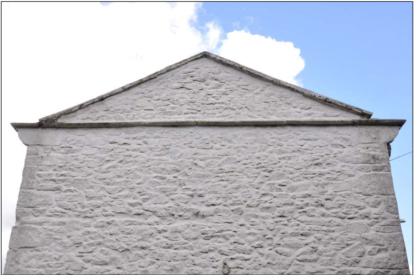
Photo 6: Detail of tabling and kneelers in south-west gable
