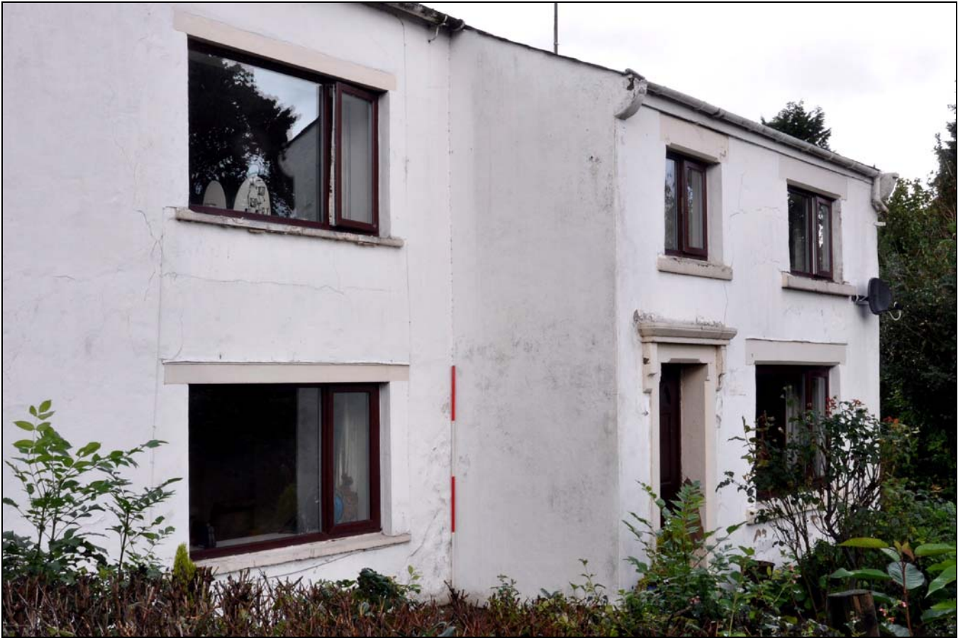
Photo 4: Front of house, with 20th century windows in part of former barn at left
