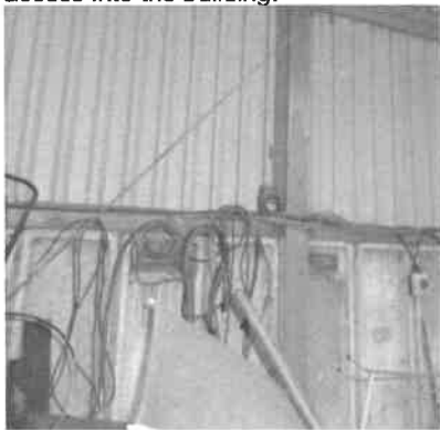
the internal view of the walls.
