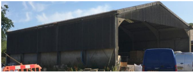
Concrete portal building front and side
