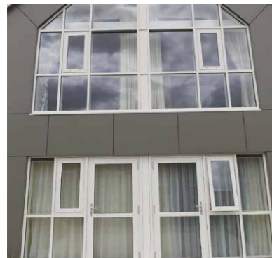
Aluminium Curtain Walling to feature gables
