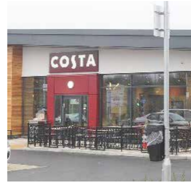
Red Cladding & Aluminium Glazing system
