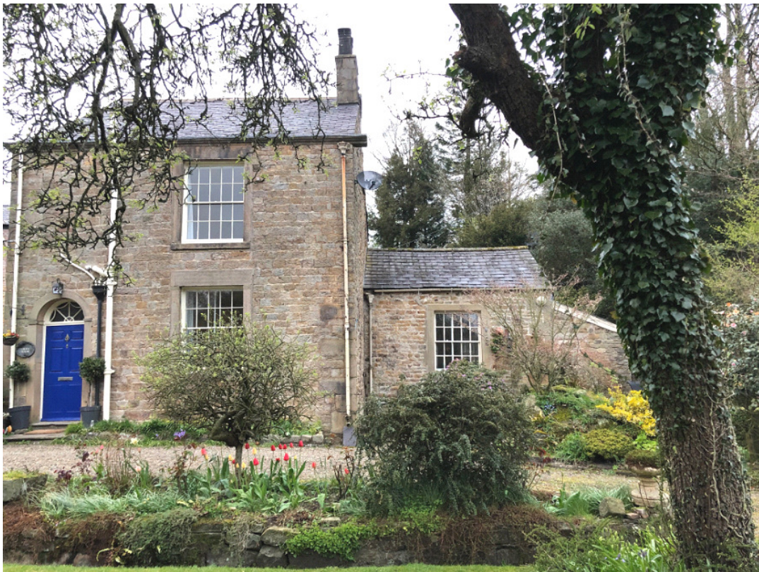
Photograph 1: Grove House (front elevation)
