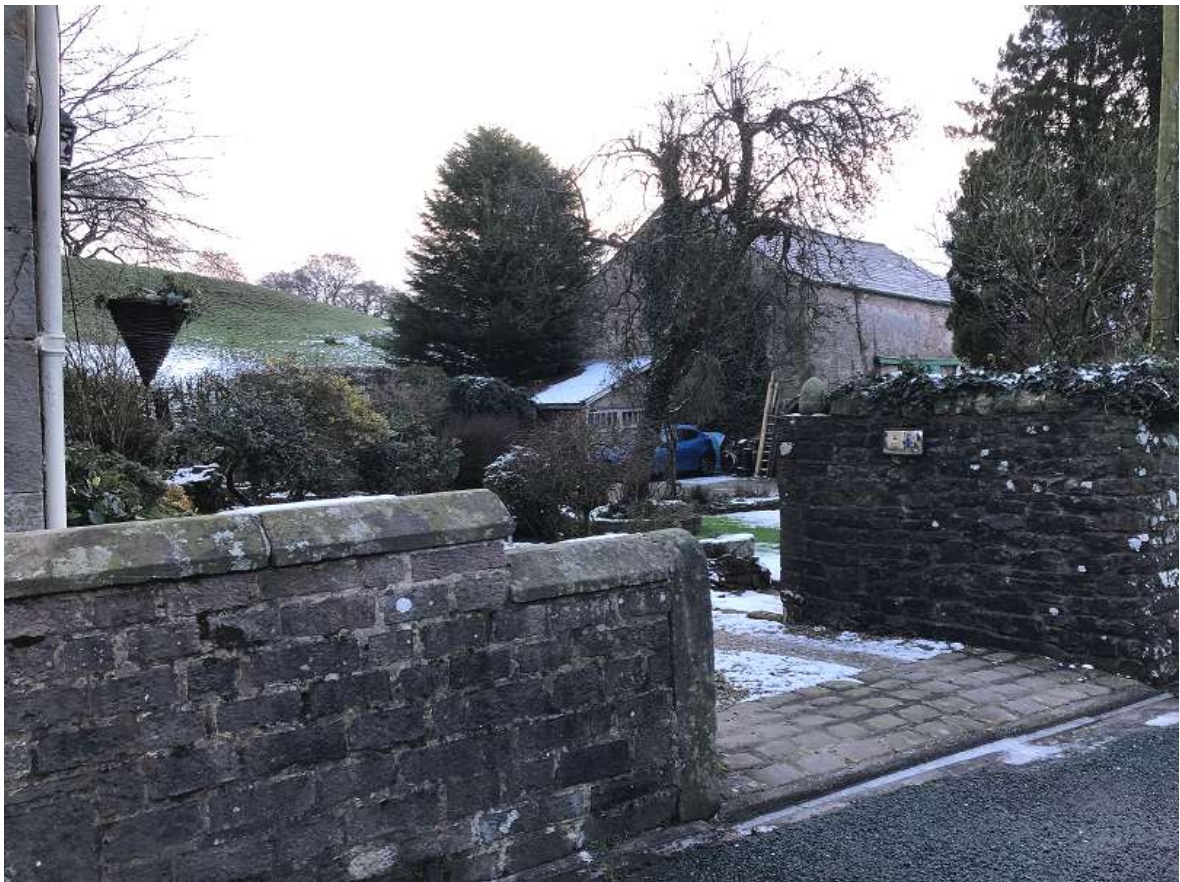
Photo a) Current view from Malt Kiln Lane of the lean-to-style garage attached to Kirk Mill's C19th Barn with Leagram Farm fields adjacent to the garden.
