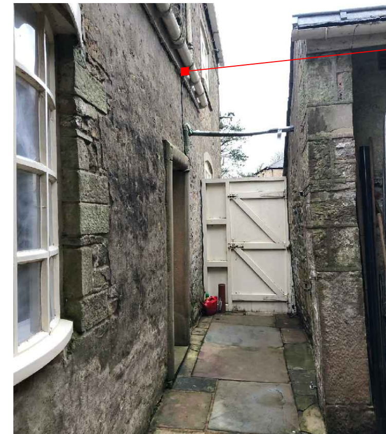
EXISTING DWELLING SHOWING GUTTERING POSITION OF KITCHEN Scale NTS
