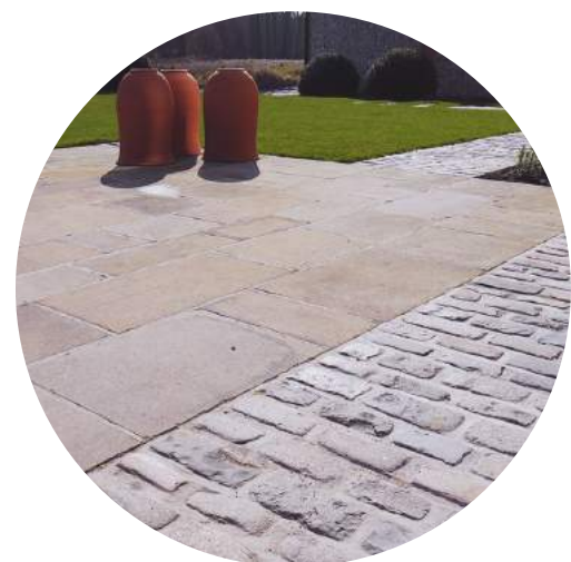
Stone flag and setts hardstanding
